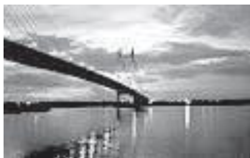
Second Hooghly Bridge(Illuminated)
