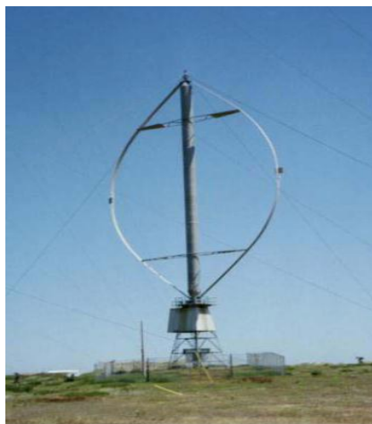
Figure 12: VAWT (Darrieus type) for electricity generation
