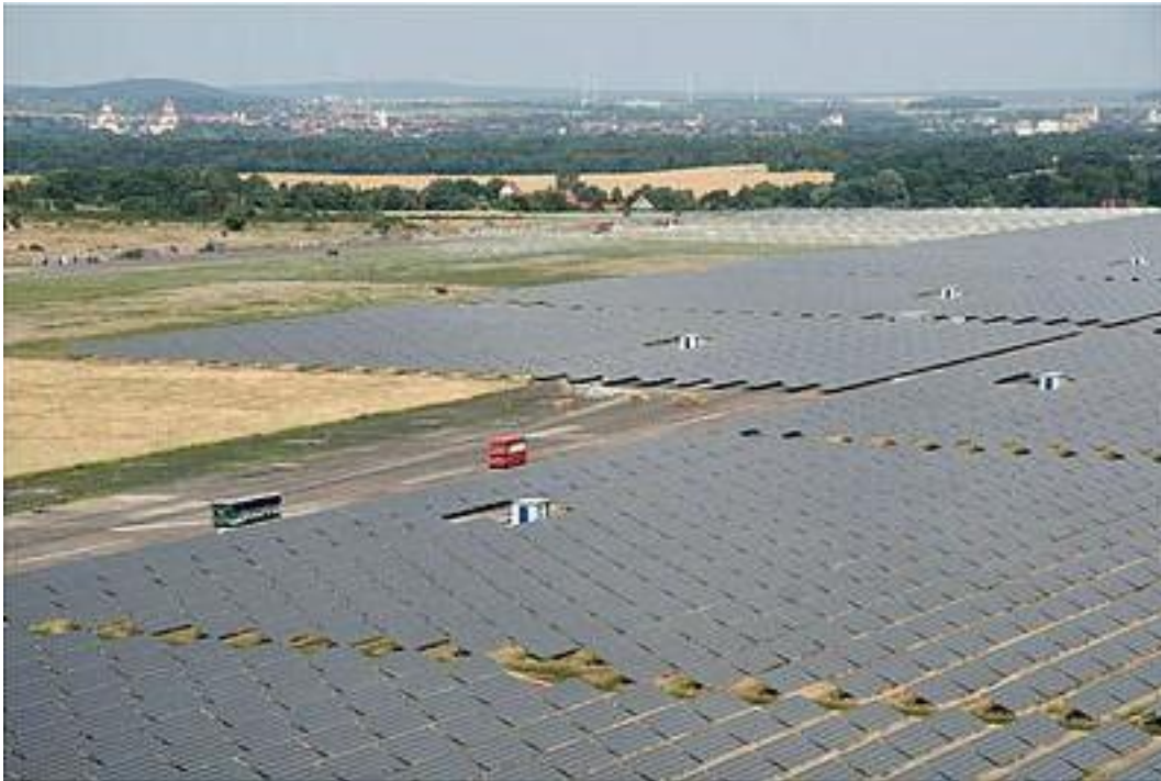
Fig. 9 – First solar 40 MW CdTe PV array installed in Germany, consisting of 550,000 solar thin film modules from cadmium telluride which supplies about 40 000 MWh of electricity per year.
