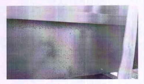
there is lot of dirt and dust over the solar panels. This reduces the efficiency of Solar Plant, it should be cleaned on daily basis...
