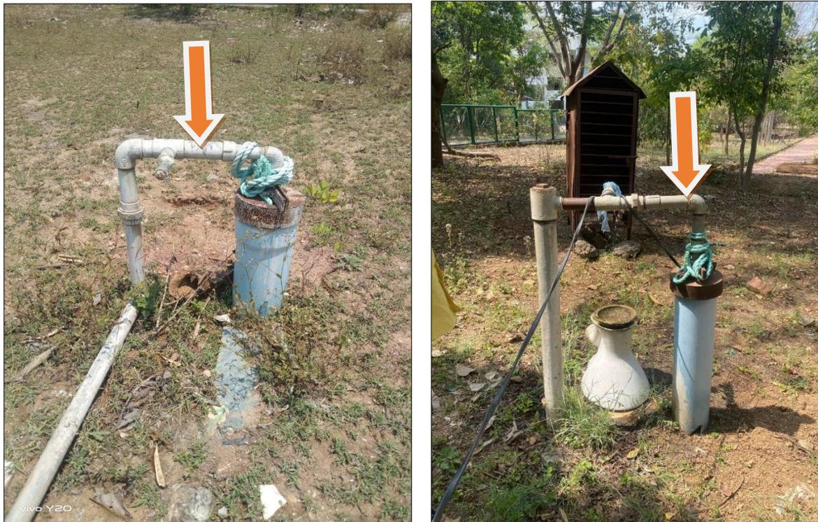
Figure: - 2.3 Requirement of water meter on bore well
